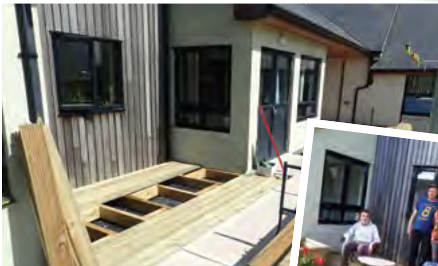
Work is well underway – learners on lunch break!
